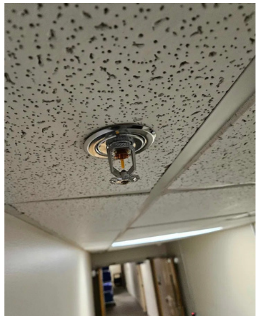
Clean Sprinkler Head (Correct)
